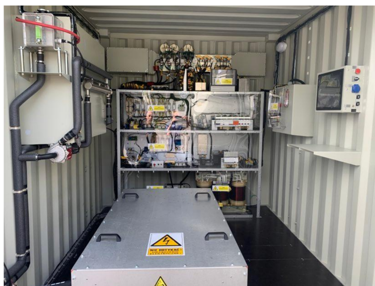
Figure 5. DC/AC converter for conversion converting trolleybus 600 V DC overhead line voltage into a 400 V AC commercial standard (operating in Gdynia, Poland; the battery-based energy storage is in the box placed on the floor).
