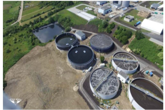
FIGURE 6. Biological part of the WWTP in Swarzewo [64].
