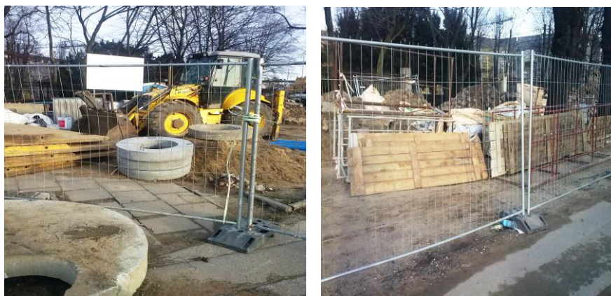
Fig. 1. Examples of elements of the building site and site compound protected in a reckless and inappropriate manner
