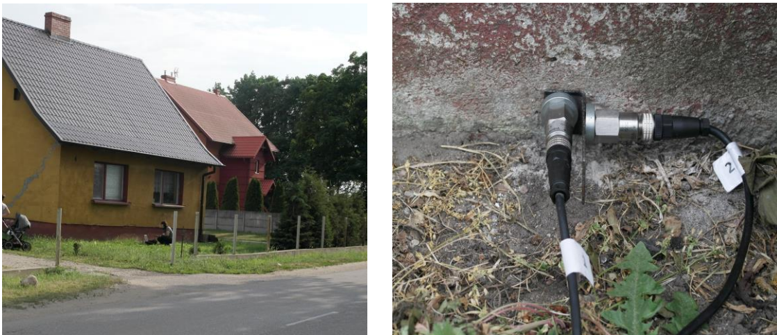
Fig. 1. Example of a building subject to vibration measurement tests (on the left), sensors installed on the wall near the ground level (on the right)
