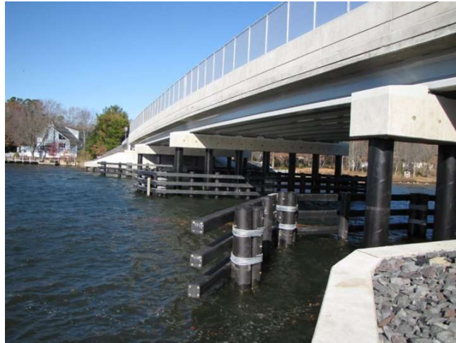
Fig. 4. CFFT piles protecting the intermediate supports of the bridge in Lacey Township, NJ, USA [7]
