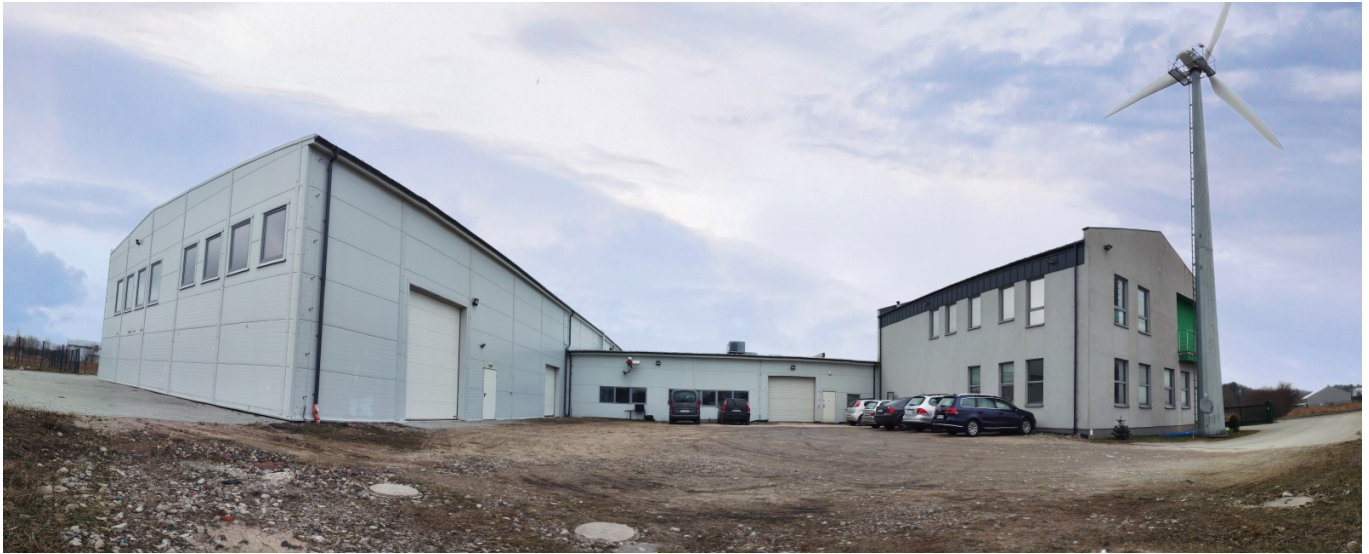
FIGURE 2 - The headquarters of the technology company MMB Drives has its own power sources in the form of a wind farm, photovoltaic panels, and a heat pump.
