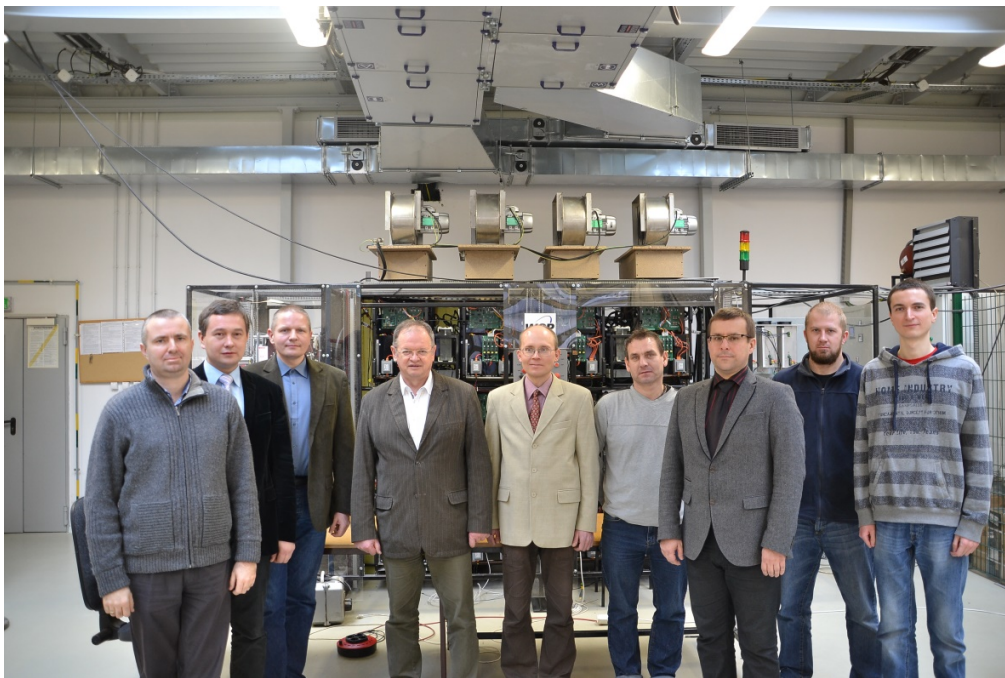
FIGURE 1- Prof. Krzeminski's university collaborators and mentees on the world's first prototype of a medium voltage power electronic transformer for the oil & gas industry [1]
