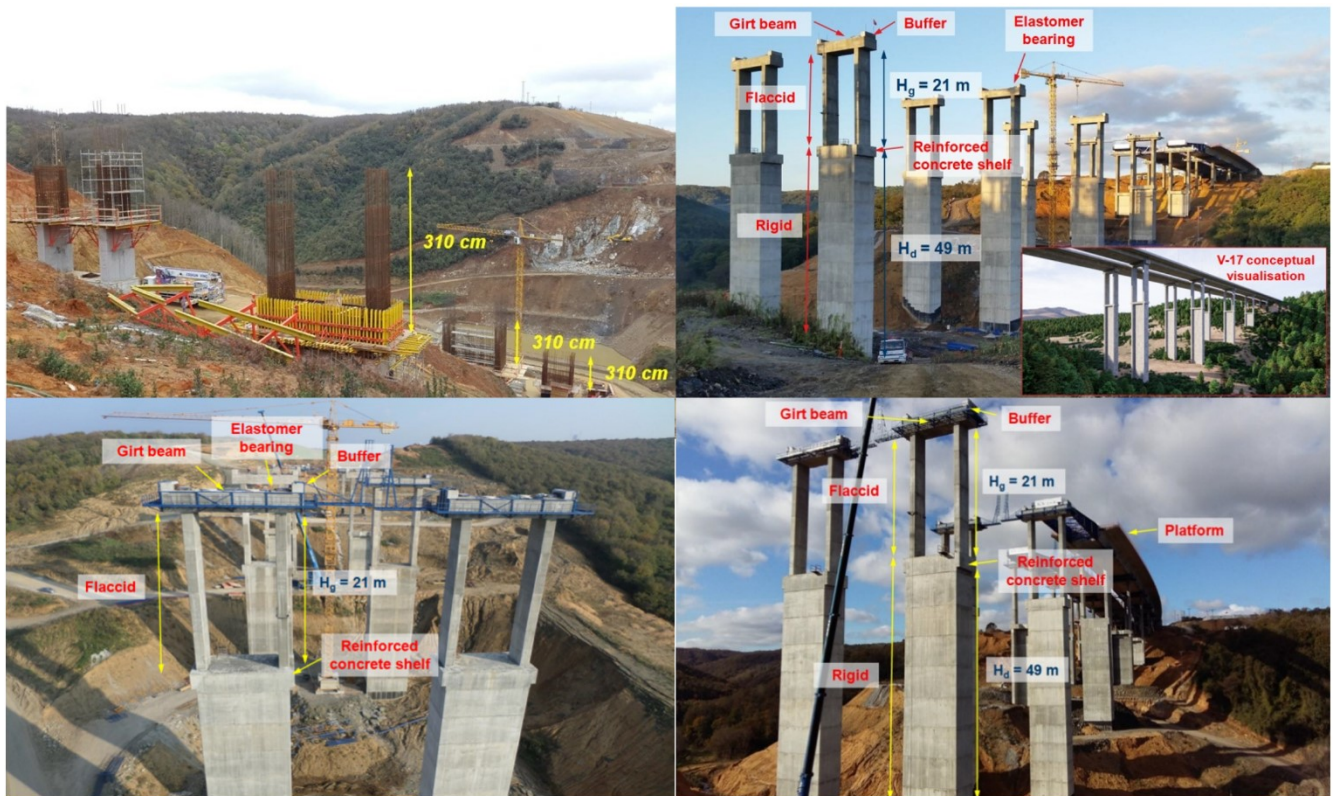
Figure 5: Photos from the implementation of the new DDC2 algorithm on the Northern Marmara Highway construction site
