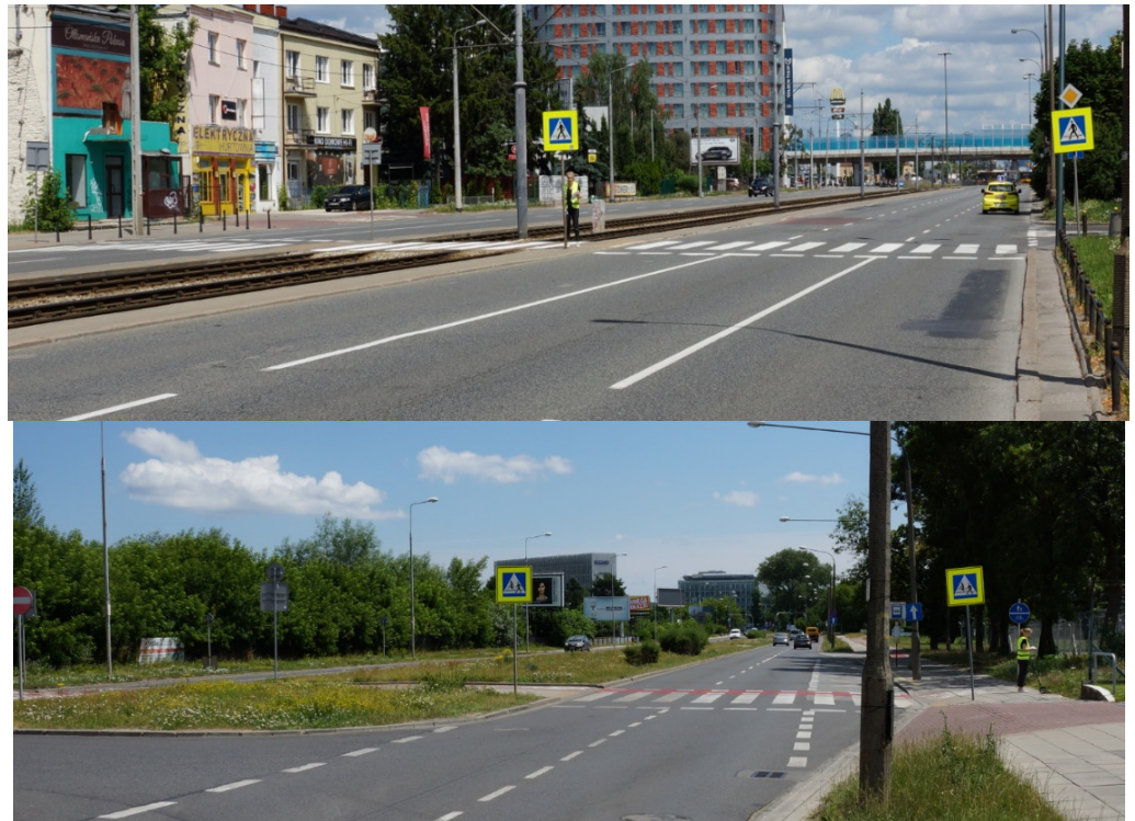
Figure 1. Examples of pedestrian crossings on 2 × 2 and 2 × 3 cross-sections in Warsaw, with no additional treatment.
