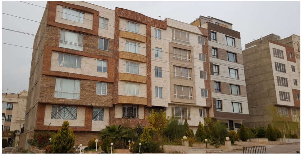
Fig. 1 Newly constructed adjacent buildings without sufficient SD, and with different base and floors levels (Qazvin, Iran)
