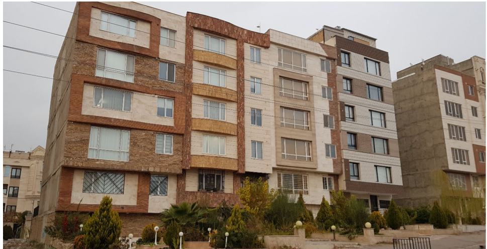
Fig. 1 Newly constructed adjacent buildings without sufficient SD, and with different base and floors levels (Qazvin, Iran)
