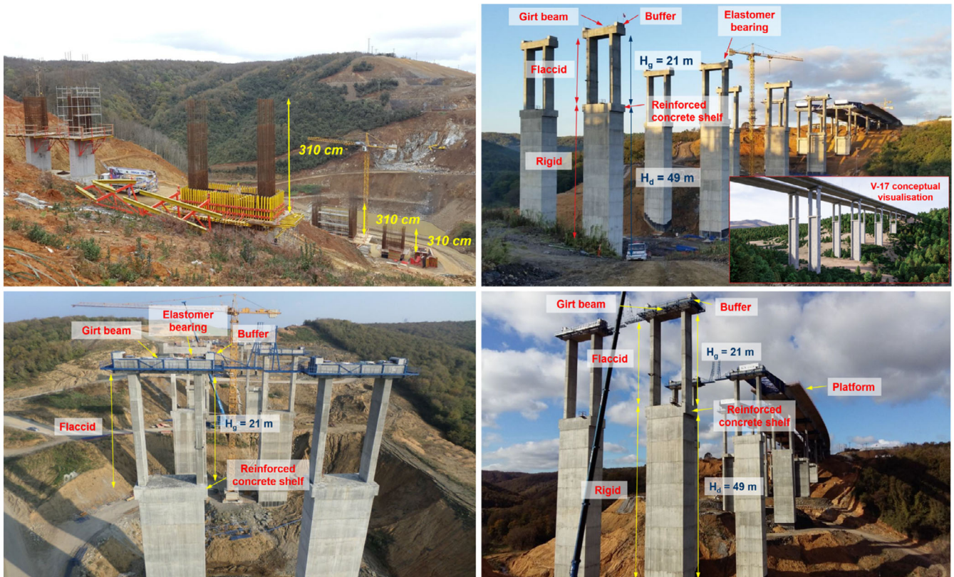
FIGURE 24 Photos from the application of the new DDC2 algorithm on the Northern Marmara Highway construction site
