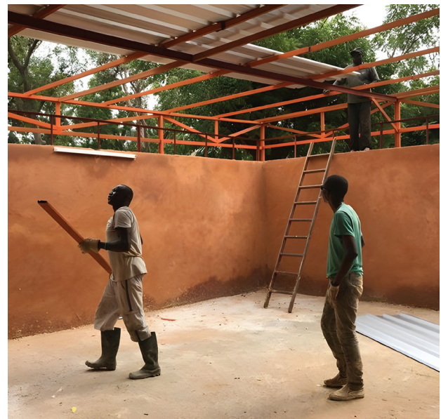
Fig. 7. Primary School, the Quartier Dixième, Thiès, Senegal. Roofing structure (source: image courtesy Let's build my school – humanitarian organization)
