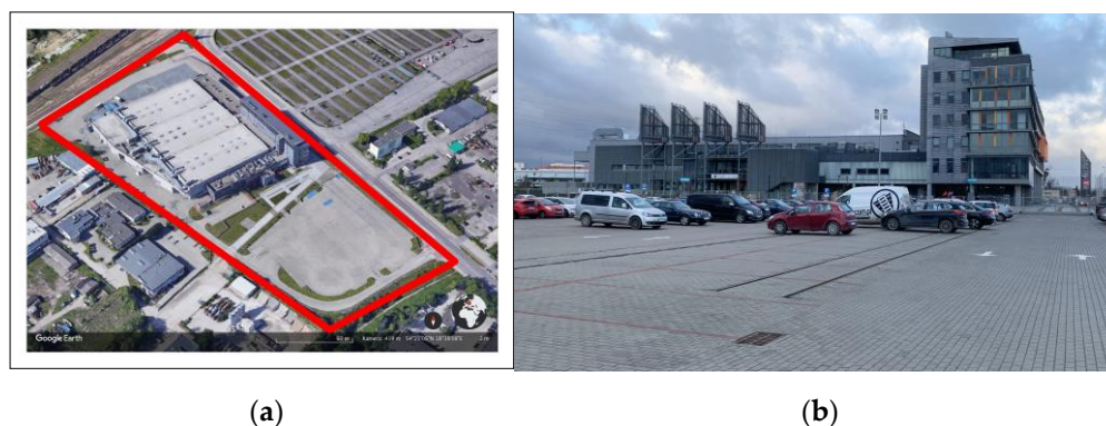
Figure 1. (a) Location and development around the Gdansk International Fair building in Gdansk, Poland (source: Google Earth). (b) View of the MTG entrance area (photo: Agnieszka Gebczynska-Janowicz).
