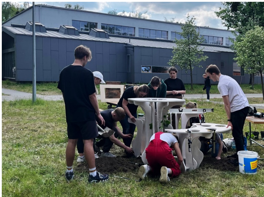
Figure 12. Assembly of the structure.
