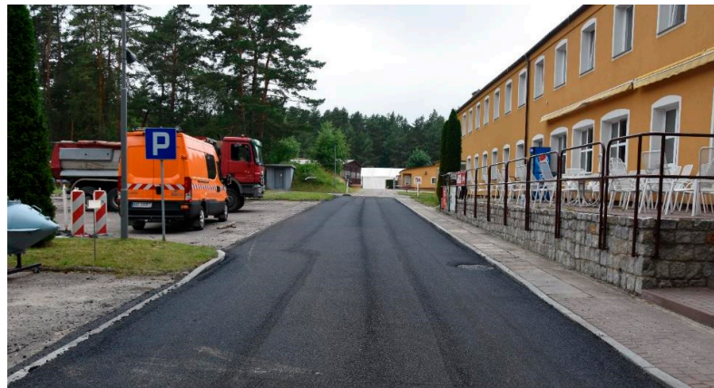
Figure 9. First long test section (D)—Dąbrówka, June 2019.
