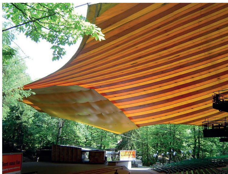
Fig. 3. Roof of the Forest Opera in Sopot (2009).
