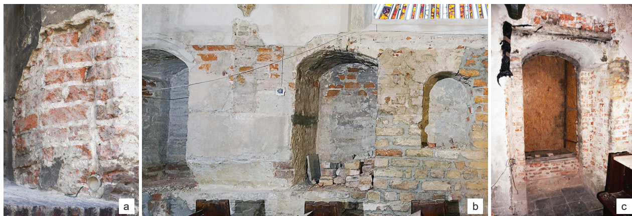
Fig. 4. Discoveries in the northern wall of the chapel at St. Joseph's Church in Gdańsk:
