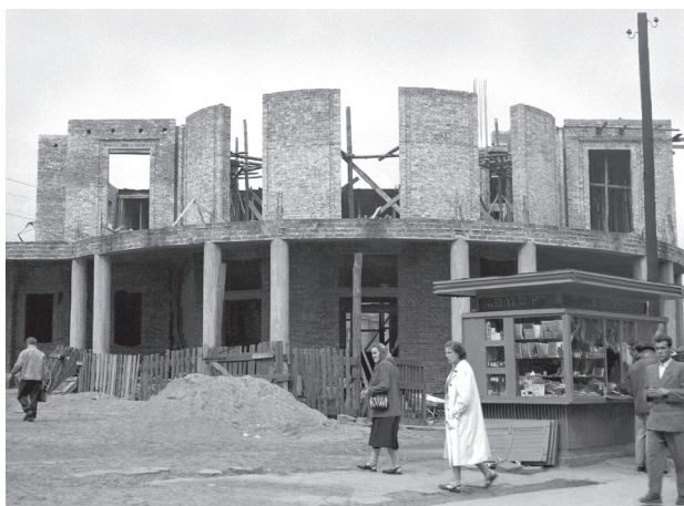
Fig. 2. The new building of the electric railway station in Gdynia under construction, 1958 (KFP) (photo by Z. Kosycarz)
