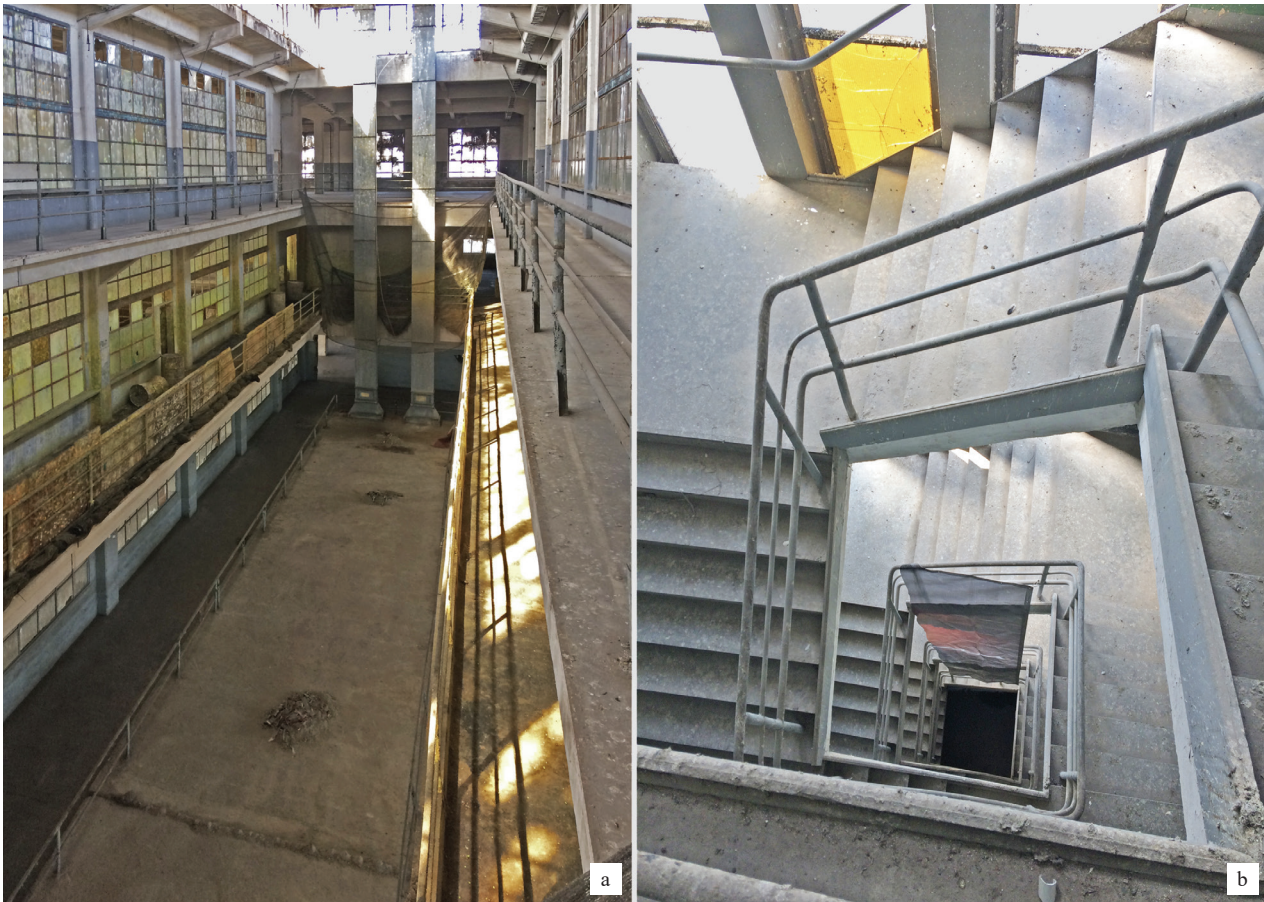
Fig. 6. Interiors of the Main Warehouse (89A), so-called the U-Boat Hall, 2019 (before the start of conservation works): a) repetitive floor of the building (6 th floor) – top view of one of the atriums, b) the staircase – stairs in all three staircases – double L-shaped stairs, monolithic, reinforced concrete structure (photo by A. Orchowska-Smolińska)
