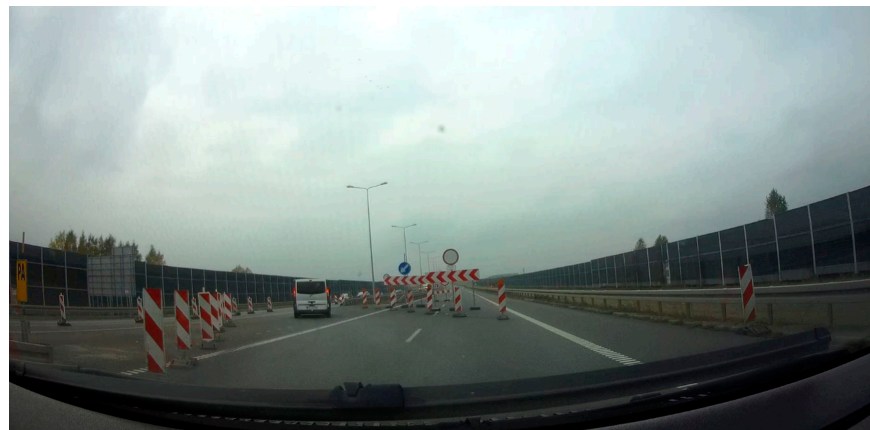
Figure 5. Example of a recorded event—unexpected road works.
