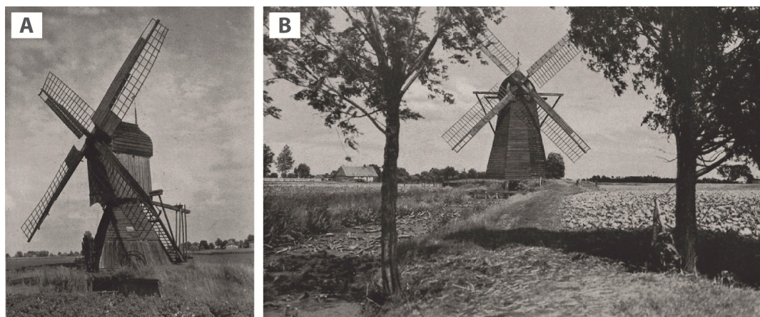
Figure 5. Drainage windmills from the Vistula Delta (Zirkwitz 1938, 72), A: Hollow post mill, B: Tower mill.
