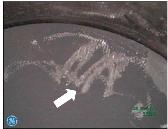
d) Piston crown – thick layer of soot, identification numbers not visible (visible trace after moving the video endoscope probe)
