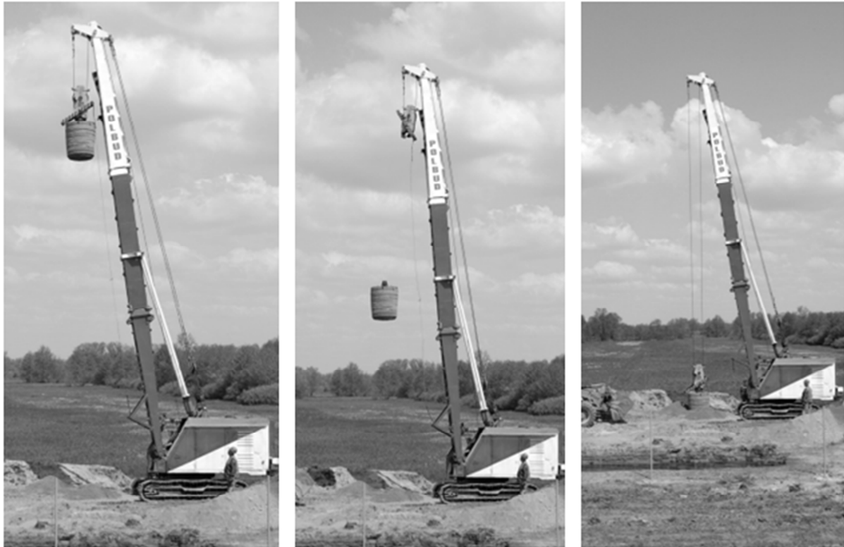
7. Dynamic soil compaction, A2 motorway section Koło-Dąbie (own photo)
