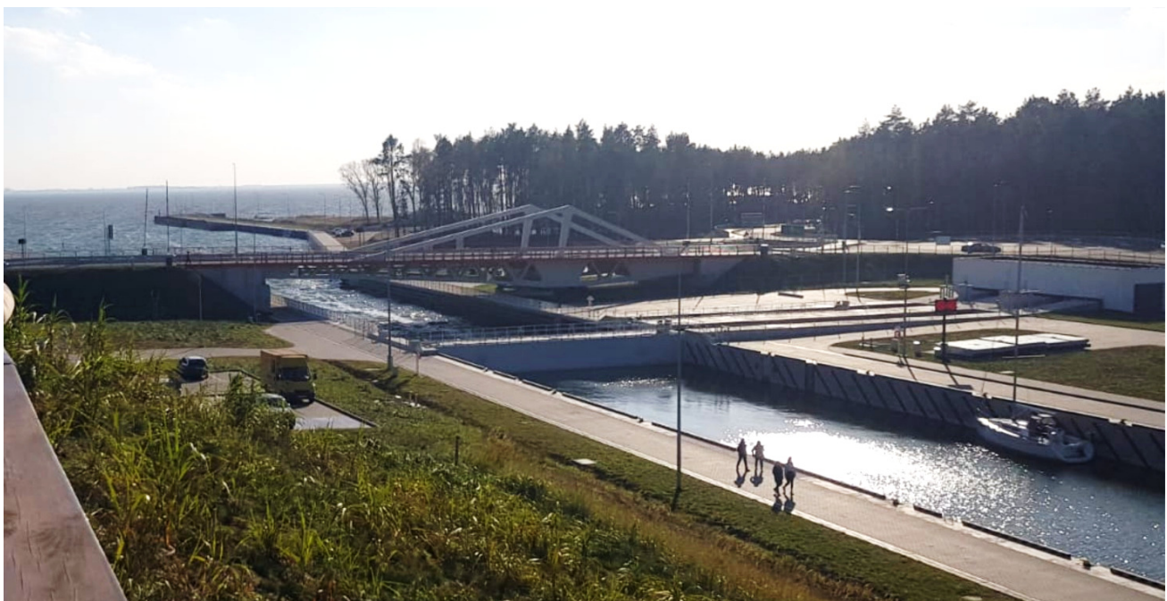
Figure 4. Current view of the Vistula Spit channel.
