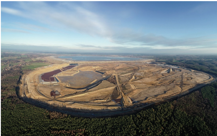
Fig. 1. The Żelazny Most tailings storage facility (OUOW) with the South Headquaters under construction – the main building of the Hydrotechnical Department
