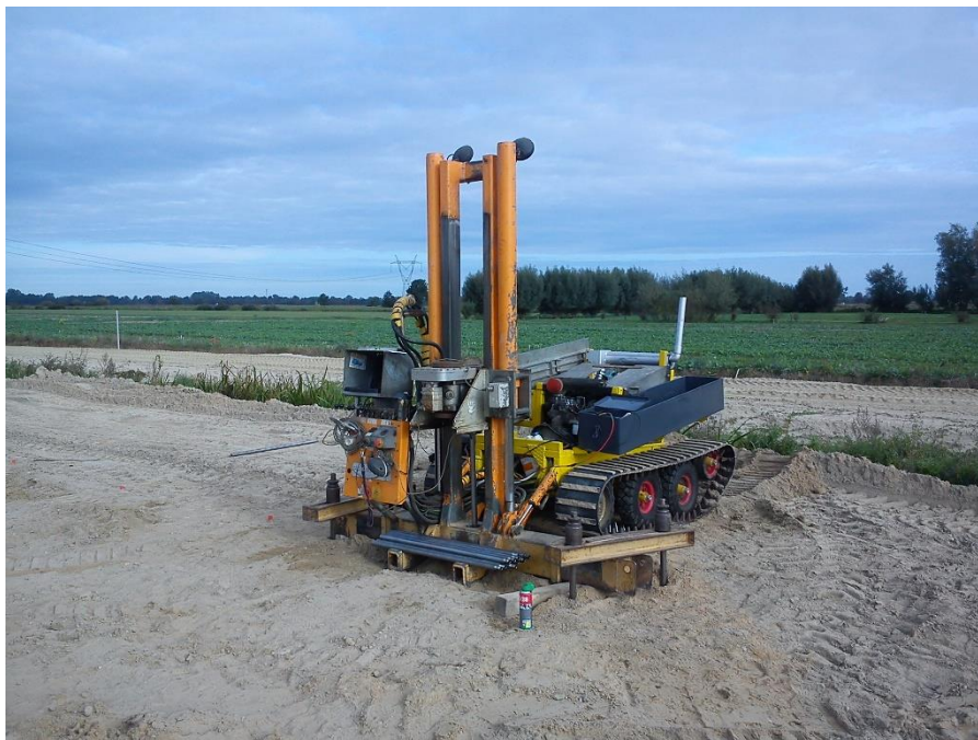
Photograph 4.1. Testing site (author: Jakub Konkol)
