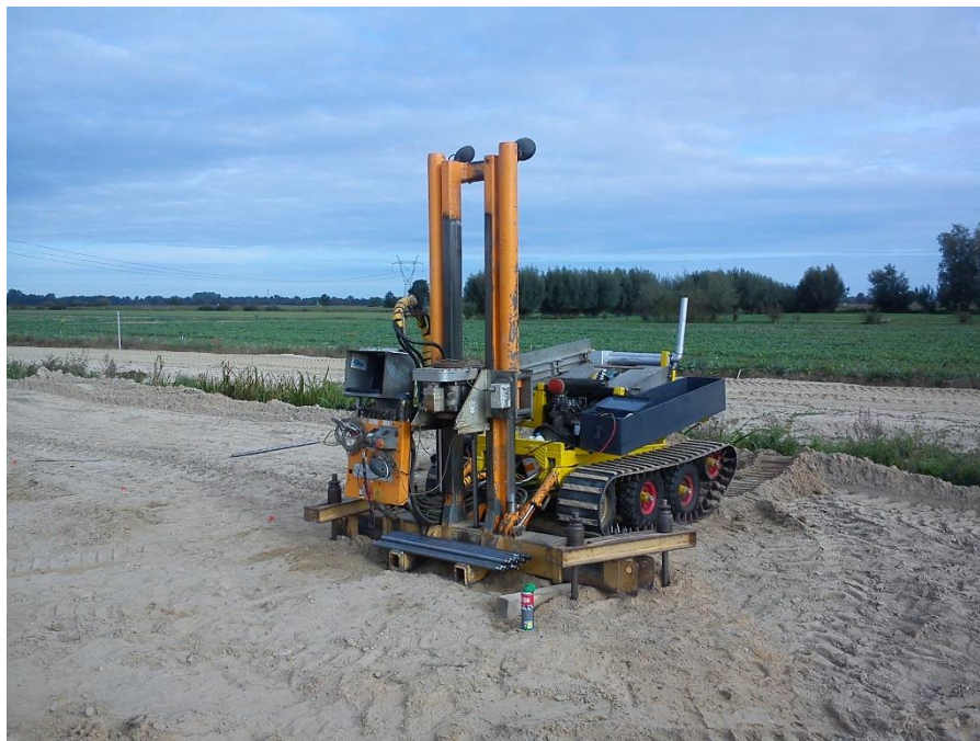
Photograph 4.1. Testing site (author: Jakub Konkol)
