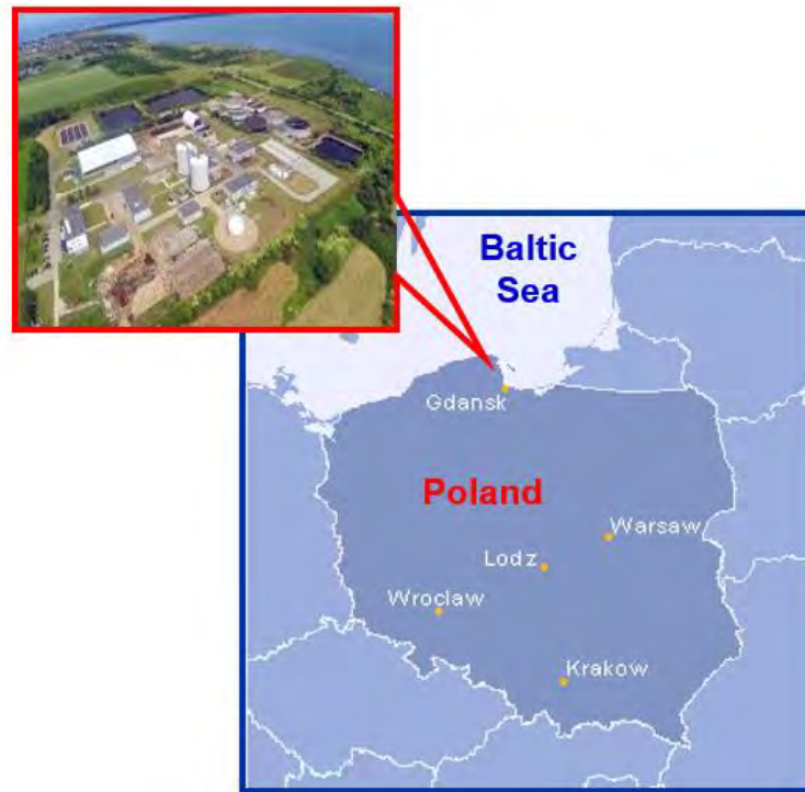
Figure 7- Swarzewo WWTP in Swarzewo, Poland
