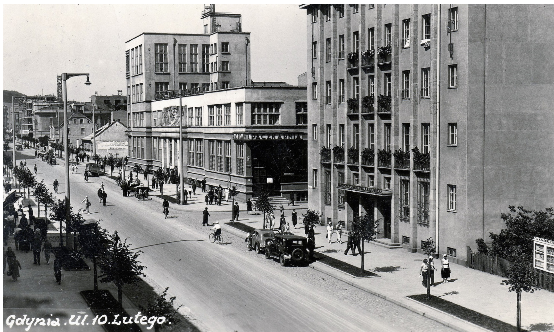
Fig. 1. Gdynia, 10 Lutego Street, the arrangement of the street in the second half of the 1930s; photo from private archives.
