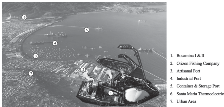
Figure 4. Bay of Coronel and Bocamina I & II, April 2018.
