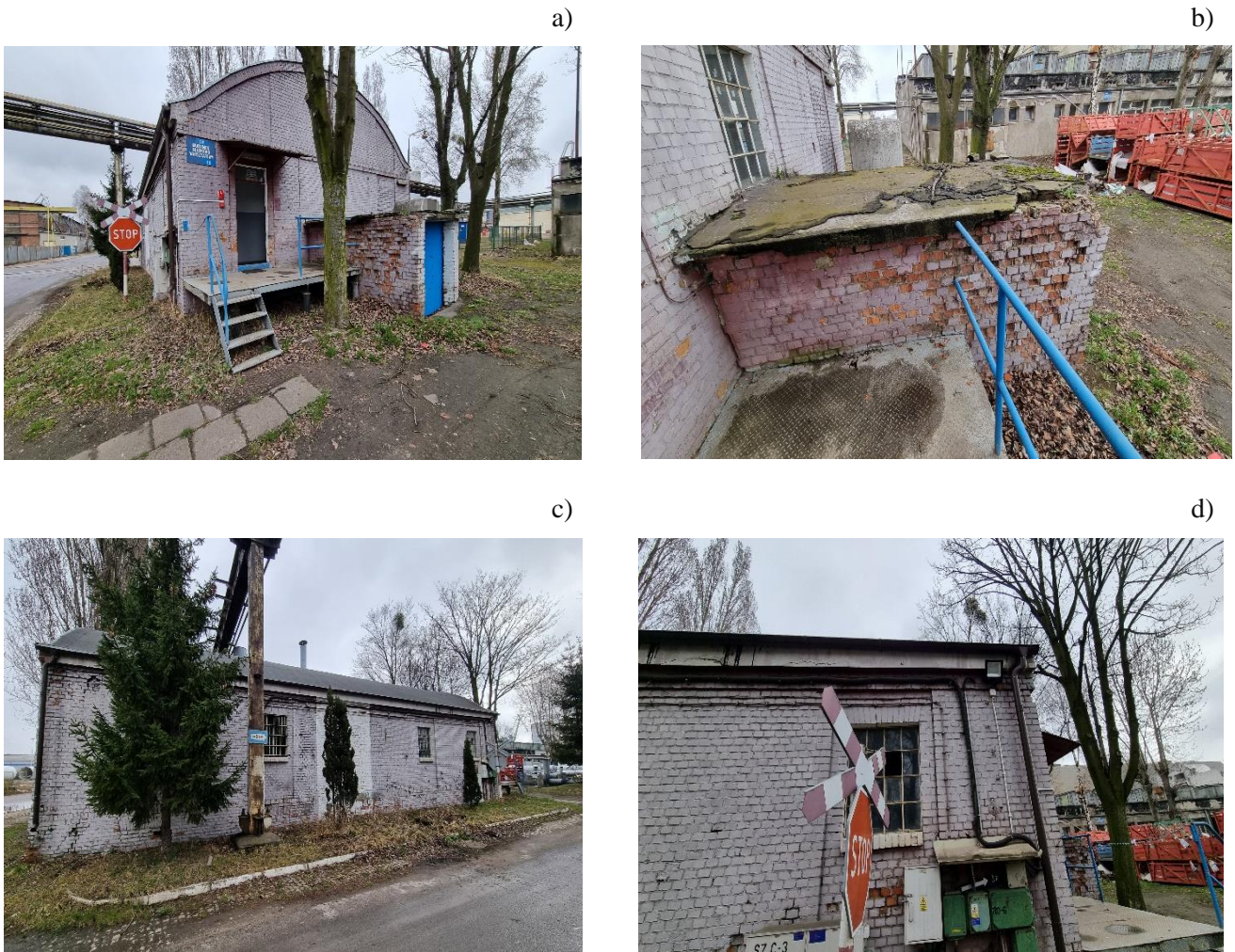
Photo 2. Warehouse building - elevations: a), b) south-eastern, c), d) south-west
