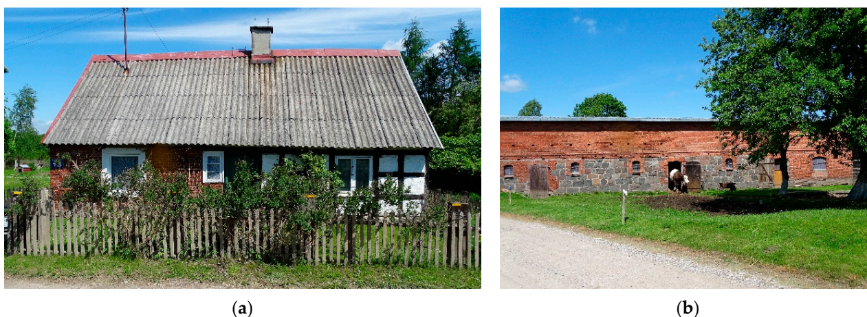
Figure 3. Historic farm buildings in the study area: (a) a house of mixed construction (of brick, half-timbered) with a high, steep roof; (b) a cowshed of brick and stone with a semi-flat roof (photos by A. Górka).
