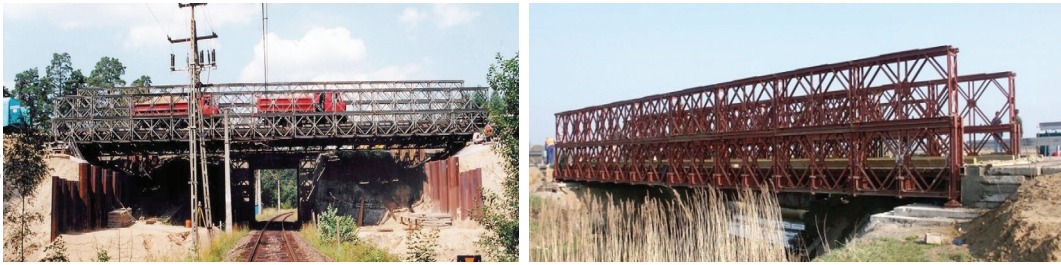
Figure 2. Diversion road with MS 22-80 bridge
