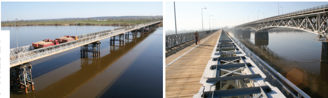
Figure 3. DMS-65 detour bridge, Chełmno, Poland
