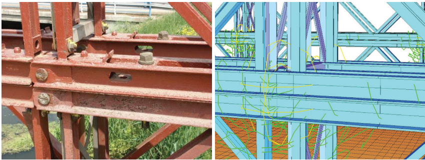
Figure 4. Detail of bolt and screw connections between lattice segments and 3D FEM visualization with GAP elements used to connect between segments in a Bailey-type panel
