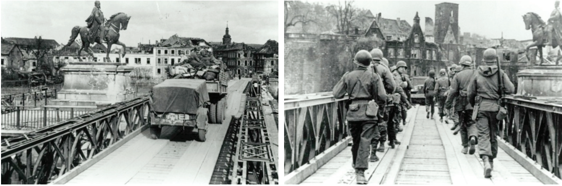
Figure 1. Application of Bailey bridges during WW II (70th Infantry Division Association, n.d.)
