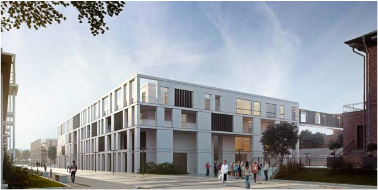
Figure 1: Eco-Innovation Centre, Gdańsk University of Technology, Gdańsk, Poland. Authors: FORT Taraszkiewicz Architekci Sp. z o. o. in Gdańsk, Poland.
