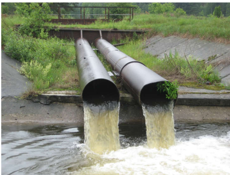
Figure 2. Discharge of brown coal mine waters treated in settling ponds.
