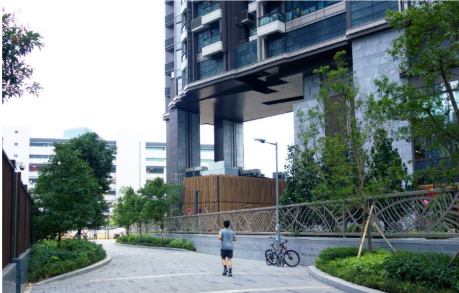
Fig. 4. The Kai Tak Development in Hong Kong – a project, in which the design solutions for urban ventilation enhancement were applied, including open ground floor plans and building voids to facilitate air flow between buildings. Photo: Joanna Badach.
