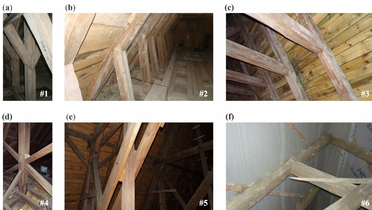
Fig. 6 Carpentry joints in church roof trusses: a Mitobądz (#1), b Pruszcz Gdański I (#2), c Kiezmark (#3), d Pruszcz Gdański II (#4), e Koźliny (#5), f Trutnowy (#6)
