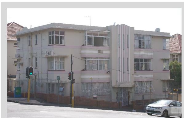
Figure 5-47 - Chelmore (527 Che Guevara Rd.) An example of the use of a flat roof in the overall study area. Limited local access to required materials made the construction of flat roofs less viable, particularly due to the increased leaking due to the lack of local expertise of installation.
