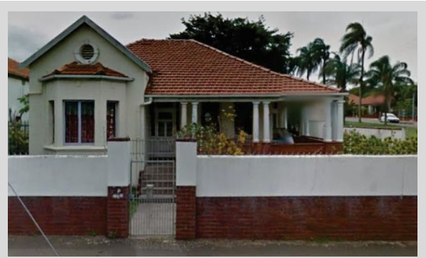
Figure 2-24 - 'Nithsdale', 2015. The overall form has been retained along with certain elements, but significant alterations have occurred. The original corrugated iron roof has been replaced with quarry tile; the timber verandah posts and ballustrades have been replaced with precast concrete columns and brick piers and walls. The finial to the gable barge board is no longer and the slightly arched timber sash windows have been replaced by aluminium versions. Most of these adaptations are due to insect or weather damage to the original timber elements, quite a common occurrence. What is also to be noted is the solid boundary wall topped with spikes and electric fencing, resulting in a significant change to the interface between the building and the street. Source: (Google South Africa, 2015)
