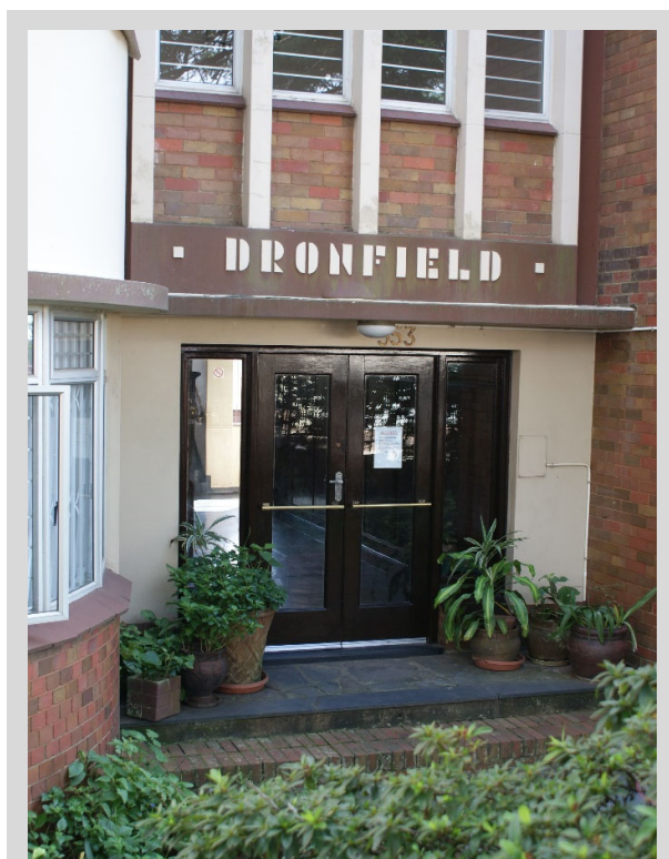
Figure 5-49 - Dronfield (553 Che Guevara Rd.) The use of face bricks of varying hues adds complexity in a subtle way to a façade. The common contemporary approach is to use a face brick of uniform colour and hue, particularly since the face brick manufacturing industry is shrinking and manufacturing processes are increasingly rationalised to produce standard batches.
