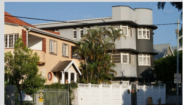
Figure 5-46 – Ashburn (358 Che Guevara Rd.) A common detail with modernist apartment buildings is to have a parapet wall facing the street and a pitched roof behind the parapet. This presents the horizontal line between building and sky synonymous with international modernist ideals while incorporating the practicality of a sheeted inclined roof in the local construction context.
