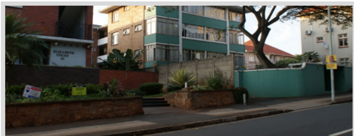
Figure 2-59 - Elizabeth Court, 31 J.B. Marks (left) and 39 J.B. Marks Rd. Elizabeth Court has implemented far less visually intrusive security measures, mainly at the building entrance, thus allowing the garden area to be visually flowing, as opposed to its neighbour that has built a solid high boundary wall topped with razor wire (that tends to rust easily in the Durban climate)
