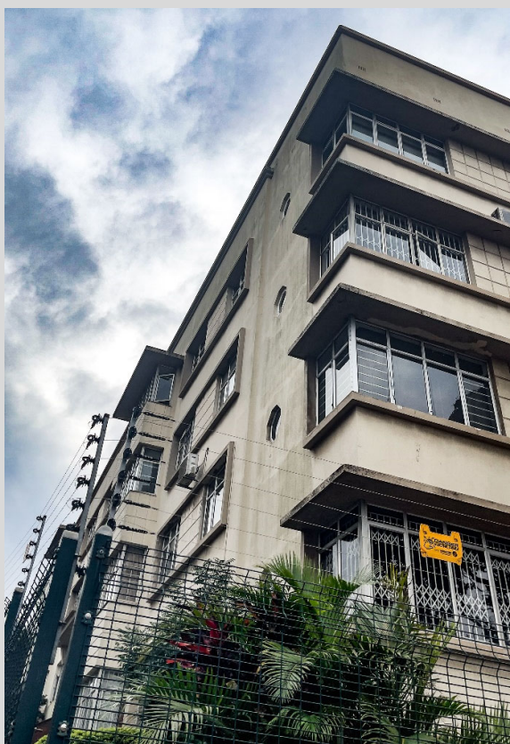
Figure 5-64 - Mount Verna (104 J.B. Marks Rd). The window treatment here contains multiple elements. The cill forms part of an overall surround to the windows and on the corner windows the lintol is expressed as an eyebrow. There are also surrounds that group windows together in defined planes, with raked plaster detailing inbetween, to add another element of variety. The original window frames have been replaced with aluminium ones.
