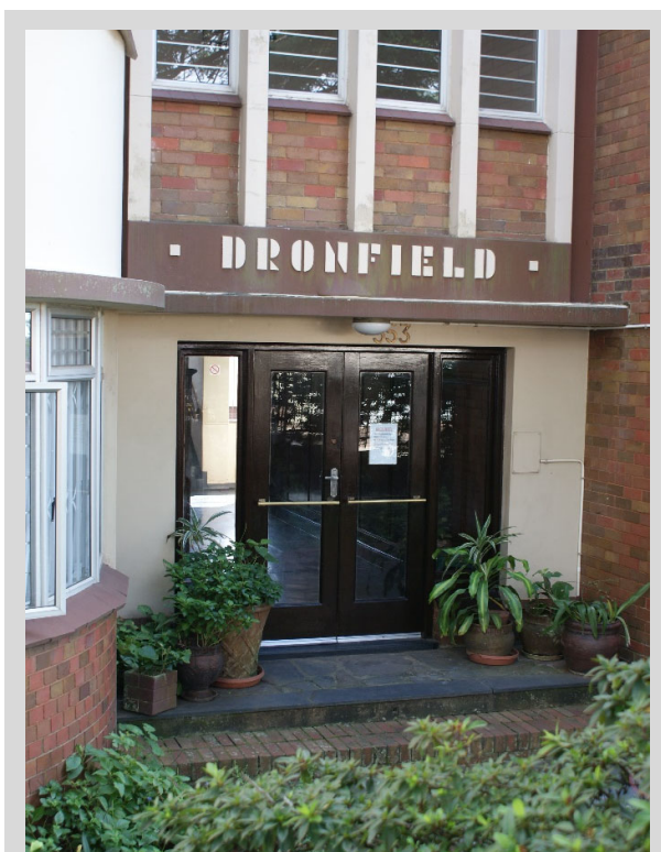
Figure 5-49 - Dronfield (553 Che Guevara Rd.) The use of face bricks of varying hues adds complexity in a subtle way to a façade. The common contemporary approach is to use a face brick of uniform colour and hue, particularly since the face brick manufacturing industry is shrinking and manufacturing processes are increasingly rationalised to produce standard batches.
