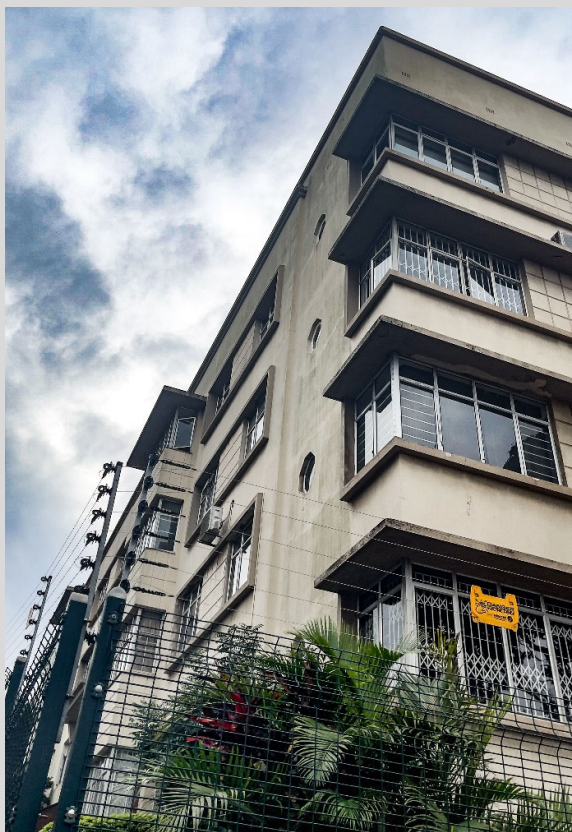
Figure 5-64 - Mount Verna (104 J.B. Marks Rd). The window treatment here contains multiple elements. The cill forms part of an overall surround to the windows and on the corner windows the lintol is expressed as an eyebrow. There are also surrounds that group windows together in defined planes, with raked plaster detailing inbetween, to add another element of variety. The original window frames have been replaced with aluminium ones.
