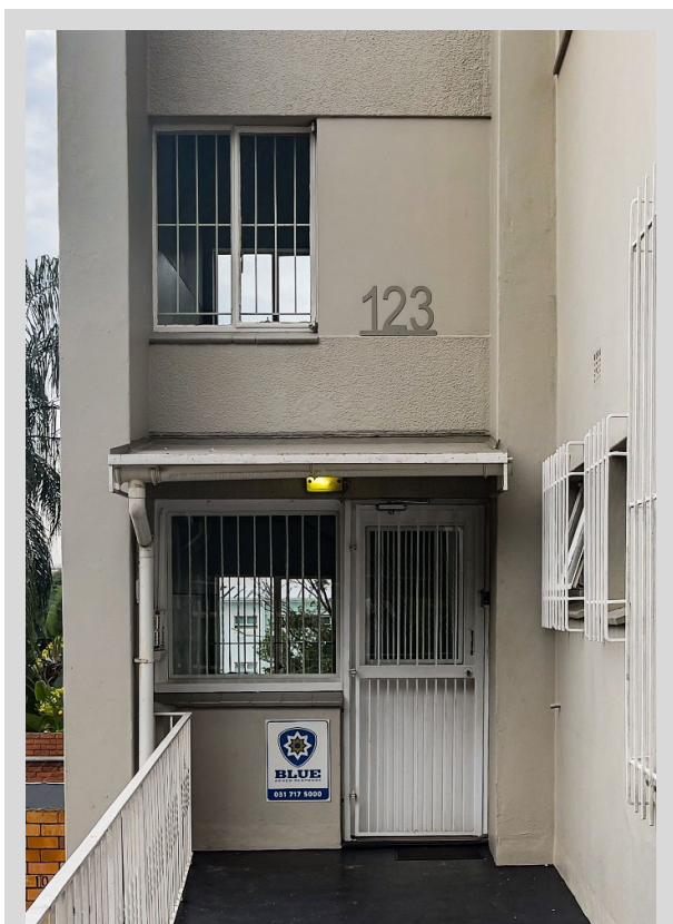
Figure 5-39 - Manning Hall (123 Lena Ahrens Rd.) Many examples exist across the study area where an additional security gate has been added to the original main building entrance door.
