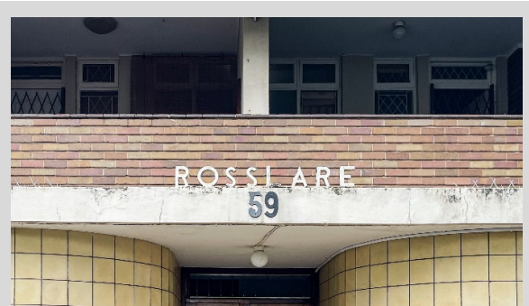
Figure 5-56 - Rosslare (59 Ferguson Rd.) The use of pre-formed lettering affixed to a wall or on top of a slab projection above the entrance is a very common element in mid-century modern apartment buildings. The lettering type (font) is also fairly consistent, with a very limited number of exceptions. The building number is an 'off the shelf' standard hardware store item undoubtedly added some time later.
