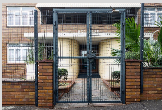
Figure 5-32 - Rosslare (59 Ferguson Rd.) Until very recently, this property had only the original low boundary wall. It featured raked horizontal and flush vertical pointing to the face brick and a quarry tile coping. The original wall has been retained with the addition of this 'ClearVu' fencing. Aside from the rather conspicuous gate frame, the overall visual disruption along the boundary is fairly minimal with this type of fencing.
