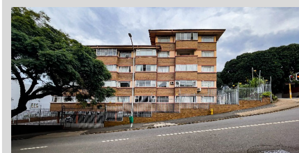
Figure 5-24 – Brierly (55 J.B. Marks Rd.) demonstrates the advantageous use of the slope. Entrance is around the corner from the top of the slope by means of a bridge, therefore an entire floor of accommodation and parking can be incorporated without exceeding the four storey height constraint.
