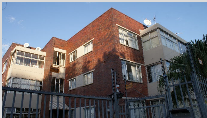
Figure 5-41 - Kenleigh (366 Che Guevara Rd.) Delineation of overall building massing is primarily achieved through the expression of 'clipped on' elements, such as the plaster finished balcony elements in this building.
