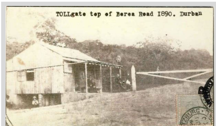
Figure 2-22 - Image from 1890 of the Tollgate at the top of Berea Rd, the road constructed in 1850 and the Tollgate constructed in 1865. It indicated the 'wooden iron' buildings (buildings with wooden frames clad in corrugated iron sheets) that were prevalent at the time in the town as an example of the more 'primitive' construction used and also indicates the thick bush in the background the covered the study area. Still prevalent in the area are houses that emulate the overall form and planning, though constructed out of brick. Currently only one 'wooden iron' structure remains in the study area (date of construction unconfirmed), located at 35 St Johns Avenue. It is secluded from most passing traffic and therefore relatively unknown. Source: (Millett-Clay, 2012)
