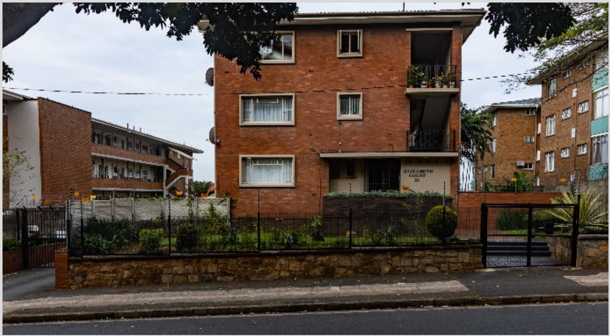
Figure 5-29 - Elizabeth Court (31 J.B. Marks Rd.) This property of 12 units with parking beneath utilising the slope typifies the average street frontage length for the study area.
