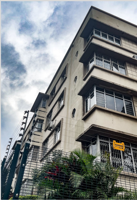
Figure 5-64 - Mount Verna (104 J.B. Marks Rd). The window treatment here contains multiple elements. The cill forms part of an overall surround to the windows and on the corner windows the lintol is expressed as an eyebrow. There are also surrounds that group windows together in defined planes, with raked plaster detailing inbetween, to add another element of variety. The original window frames have been replaced with aluminium ones.
