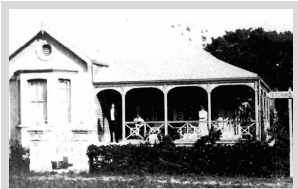
Figure 2-25 - 'Nithsdale' – 127 Teignmouth Rd, Umbilo, circa 1895. The house, though located further south than the study area, is typical of many of the single storey houses of the middle-income population of the time. Typical features are the protruding gable portion with faceted bay window, elaborately decorated ventilator and finial at the apex of the fascia; the wrap around verandah with slender timber posts and decorative brackets; the sliding sash windows with delicate mullions and slightly arching lintols; and corrugated iron roof. The property boundary was defined by hedges, demonstrating the active use of vegetation and the open visual quality to the street. Source: (Kearney, 1984, p. 75)
