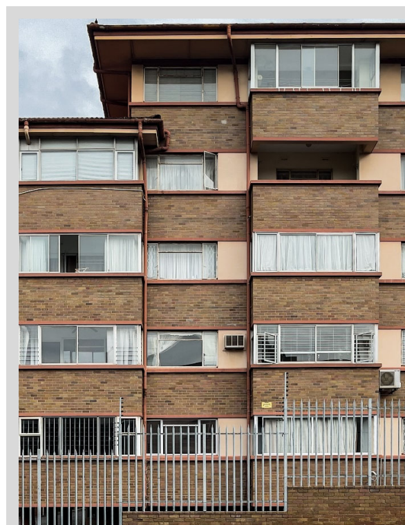
Figure 5-63 - Brierly (55 J.B. Marks Rd.). In this image only one of the balconies remain as original and unenclosed. The use of sliding windows is almost universally only found in these subsequent balcony enclosures. There is no uniformity of detailing in the enclosing, which negatively affects the perception of the visual quality.
