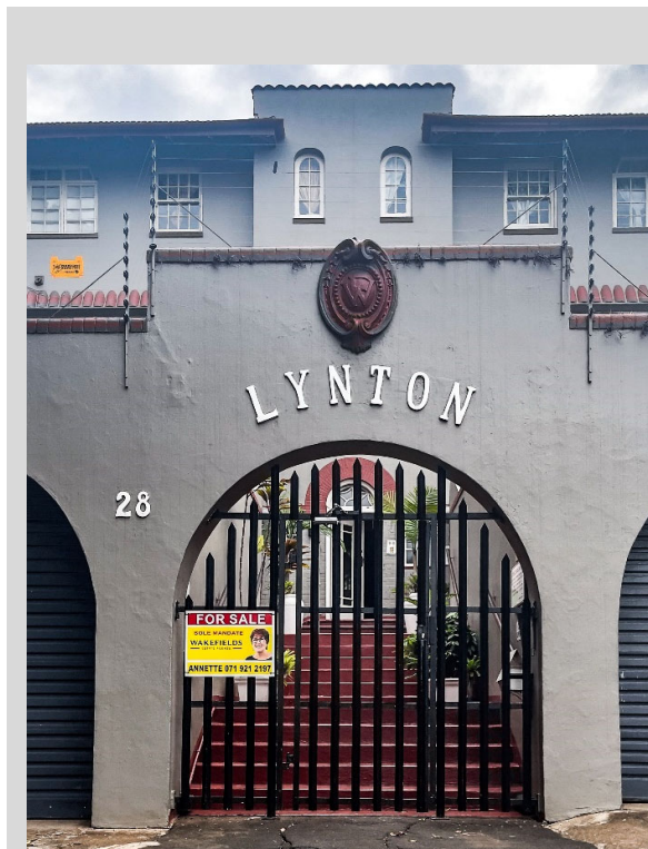
Figure 5-59 - Lynton (28 Lena Ahrens Rd.) Though somewhat obscured by the boundary treatment (which may be subsequent to the original construction), the entrance definition is enhanced by the use of an extension to the parapet wall above it in addition to the overall volume containing it sitting slightly proud to its surrounds.
