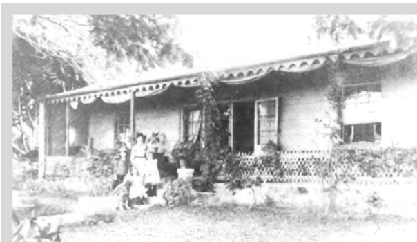
Figure 2-19 - 'Longlands' (c. 1875) is an example of the typical homes first built on the Berea. The brick and iron roofed structure with vertically proportioned windows and wrap around verandah. The canvas awnings would later translate into the bracket profiles included on later houses. Source: (Kearney, 1984)
