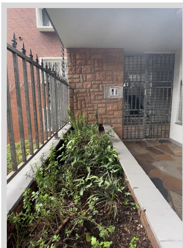
Figure 5-34 - Clayton (89 Lena Ahrens Rd.) A planter has been used along the entrance path as a balustrade, but also to add an element of variety to the streetscape and entrance experience. Until very recently, this was open with security taking place at the lobby, but now an additional gate has been added at the boundary.
