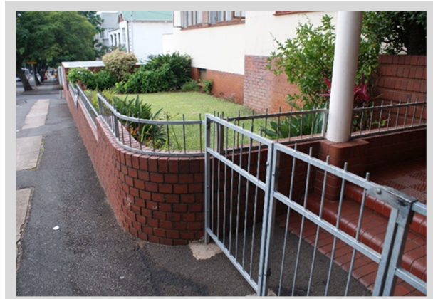
Figure 2-56 - Wynndham, ca. 1950, 408 Che Guevara Rd. This image was taken in 2019, and subsequently a higher fence has been erected. The original low brick garden wall clearly defines the property boundary. Subsequent security upgrades of a low steel railing and gate further reinforce the territoriality being expressed. This portion of garden is not easily accessed, one has to climb over the garden wall to get there. It still adds to the overall streetscape as the visual separation is minimal in comparison to the majority of properties in the area, though more compromised with the subsequent higher fence added.
