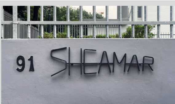
Figure 5-53 - Sheamar (91 Lena Ahrens Rd.) Here shaped metal flat bar has been used to form the building signage. The building number is an 'off the shelf' standard hardware store item undoubtedly added some time later.
