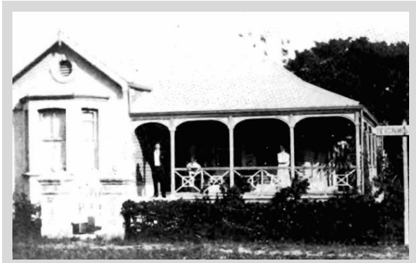
Figure 2-25 - 'Nithsdale' – 127 Teignmouth Rd, Umbilo, circa 1895. The house, though located further south than the study area, is typical of many of the single storey houses of the middle-income population of the time. Typical features are the protruding gable portion with faceted bay window, elaborately decorated ventilator and finial at the apex of the fascia; the wrap around verandah with slender timber posts and decorative brackets; the sliding sash windows with delicate mullions and slightly arching lintols; and corrugated iron roof. The property boundary was defined by hedges, demonstrating the active use of vegetation and the open visual quality to the street. Source: (Kearney, 1984, p. 75)
