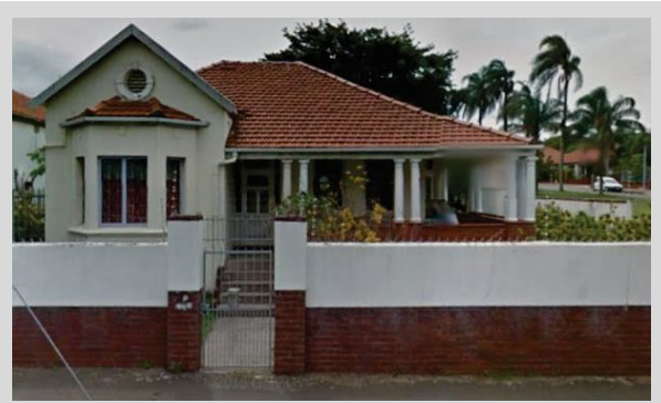
Figure 2-24 - 'Nithsdale', 2015. The overall form has been retained along with certain elements, but significant alterations have occurred. The original corrugated iron roof has been replaced with quarry tile; the timber verandah posts and ballustrades have been replaced with precast concrete columns and brick piers and walls. The finial to the gable barge board is no longer and the slightly arched timber sash windows have been replaced by aluminium versions. Most of these adaptations are due to insect or weather damage to the original timber elements, quite a common occurrence. What is also to be noted is the solid boundary wall topped with spikes and electric fencing, resulting in a significant change to the interface between the building and the street. Source: (Google South Africa, 2015)
