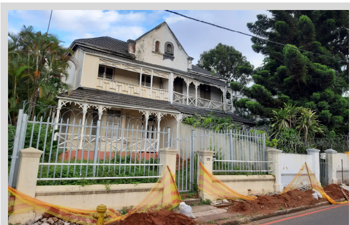
Figure 4-13 - 76/78 Hunt Rd. This 'Colonial' duplex has two units, each over two floors. In this particular instance, one unit is classified as being in a 'poor condition' as it requires a considerable amount of maintenance and this impacts on the overall building. The property ownership is usually separate for this period of construction, so it is difficult for the owner of the adjoining unit to practically influence ongoing maintenance. The formation of Sectional Title ownership addresses this shortcoming to a significant extent, though interpersonal relationships work better when there are larger numbers of owners that make up the sectional title.
