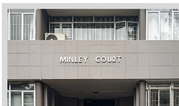
Figure 5-55 - Minley Court (138 Lena Ahrens Rd.) The use of pre-formed lettering affixed to a wall or on top of a slab projection above the entrance is a very common element in mid-century modern apartment buildings. The lettering type (font) is also fairly consistent, with a very limited number of exceptions.
