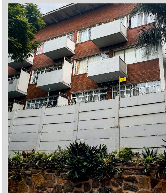
Figure 5-42 – Camberly Hall (134 Lena Ahrens Rd.) The balconies are expressed as a series of ‘prominently projecting ‘clipped on’ masses, adding dynamism to what would otherwise be a rather bland elevation.
