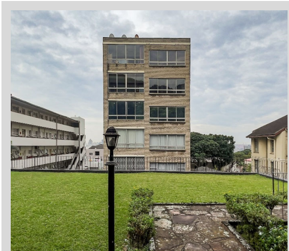
Figure 5-43 – Sheamar (91 Lena Ahrens Rd.) The elevation demonstrates what this study terms ‘mild visual density’. The overall form is singular in expression, there is limited variety in fenestration and materials. The execution is simplistic. The historic elements of the garden path and lamppost add some visual relief to be experienced from the street.
