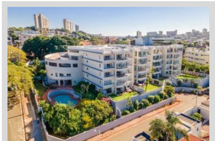
Figure 1-16 - Aerial view of a recent development within the study area. The trend of ‘drive-up’ developments (where occupants can drive up to their front door of their unit on an upper floor) is growing across the greater Berea. Source: (RE/MAX, 2022)
