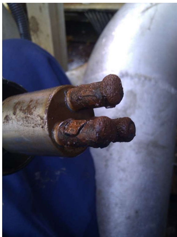
Figure 19. Condition of a sensor after 90 days of exposure to brine.
