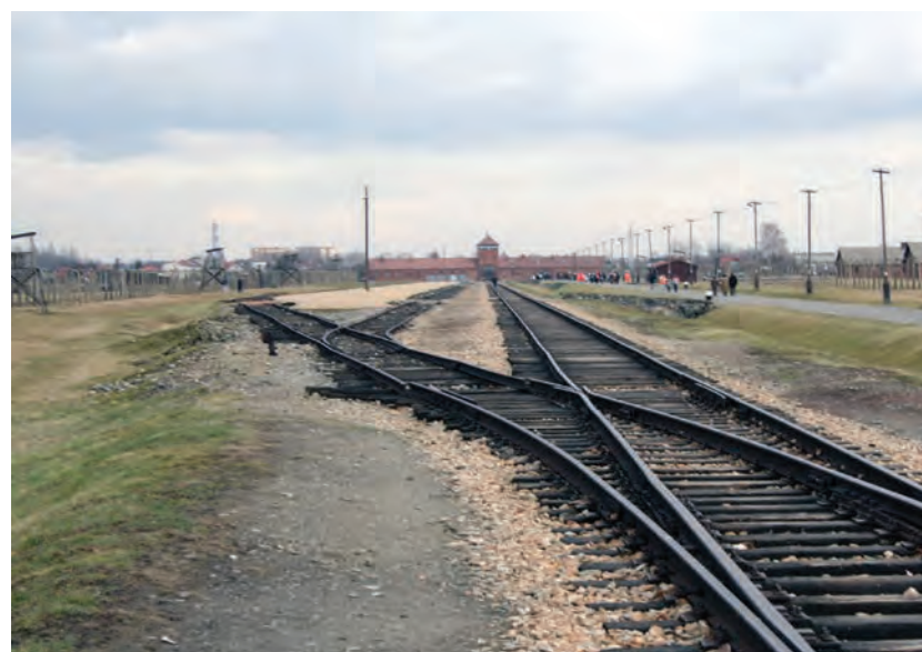
1. The railway ramp with the main gate leading to the area of the KL Auschwitz-Birkenau in the background
