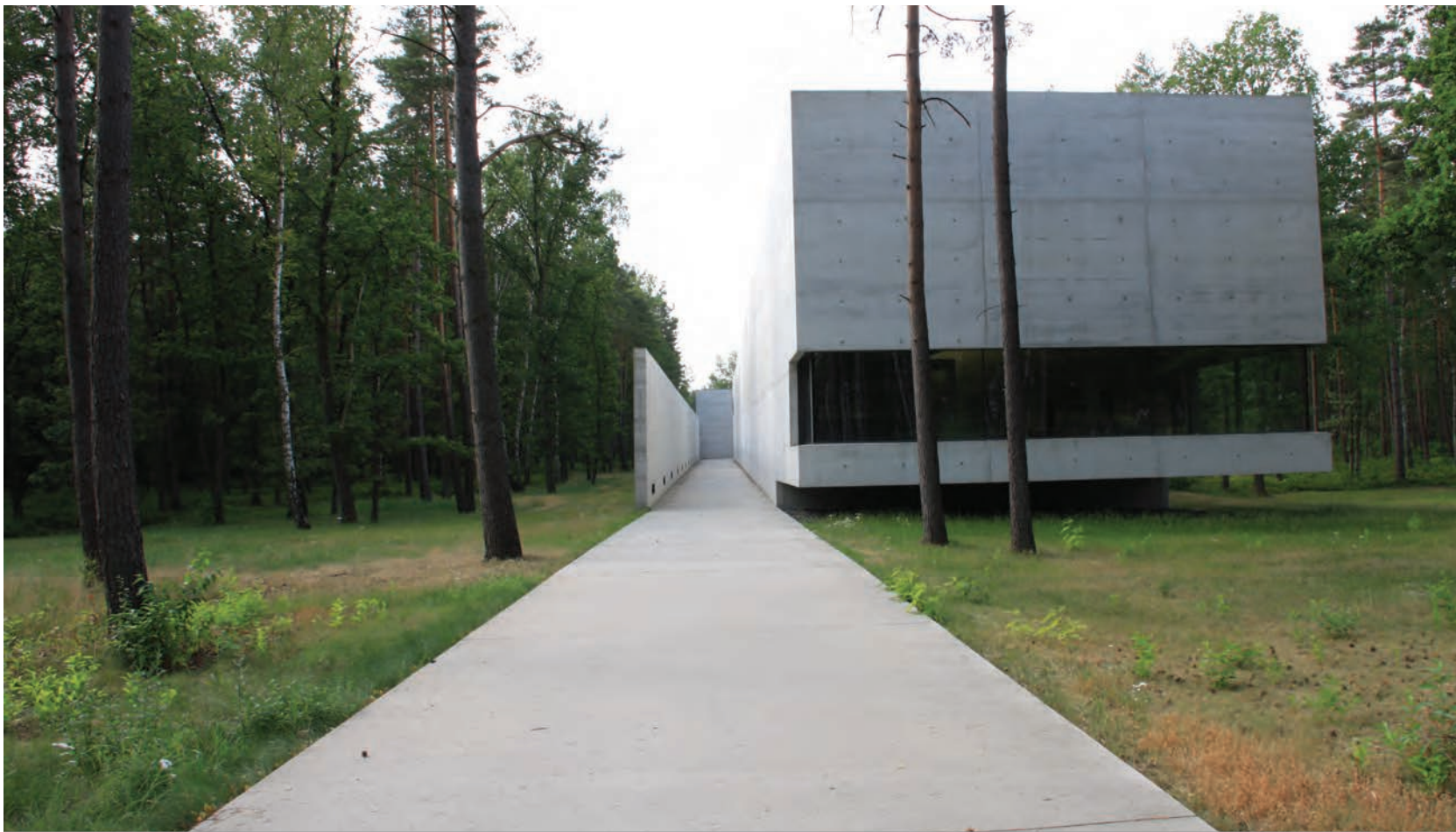
8. The overhanging part of the museum building
