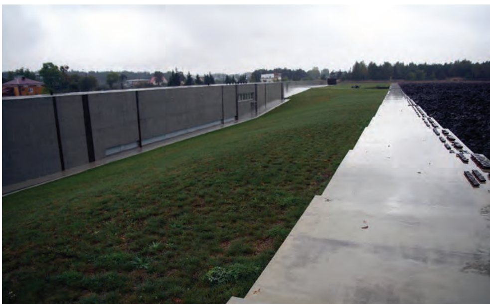
9. The museum building located on the axis of the symbolic railway ramp
