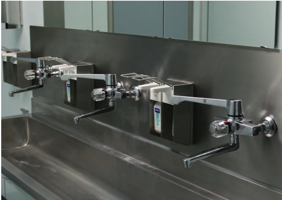
Photograph 6.3.1.5 Elbow-operated taps (an example of hygienic equipment that can be operated in a hand-contactless way); photographed by the Author, 2016
