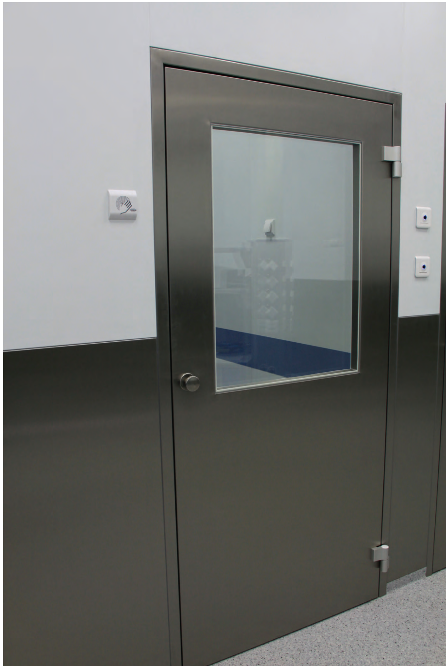
Photograph 6.2.2 Automatically opening door (a solution that reduces a possibility of contaminating medical personnel's hands); photographed by the Author, 2015
