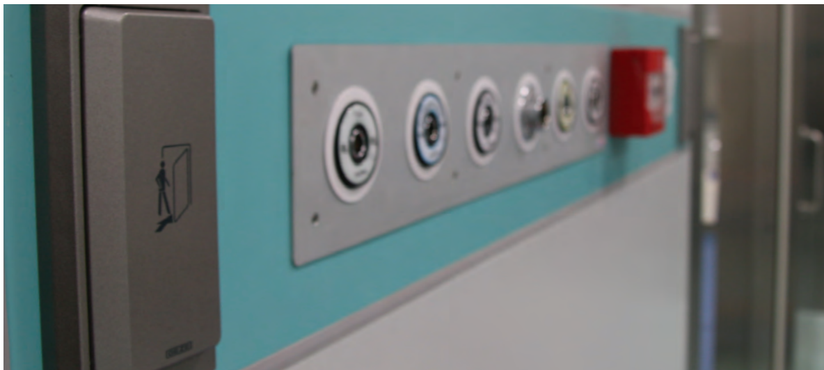
Photograph 5.5 Elements of wall finishing at an operating theatre (an example of a surface characterised by an increased resistance to disinfection procedures); designed and photographed by the Author, 2016
