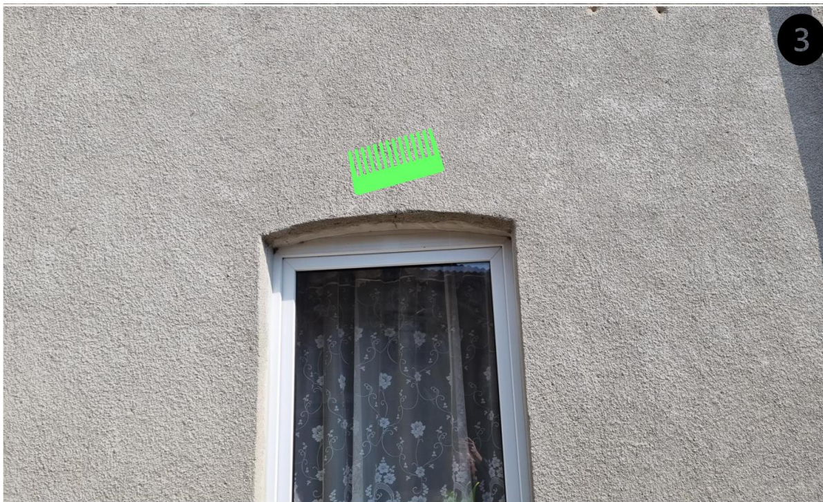
Fig. 6: Proposed location of target plates, benchmarks and feeler gauges on the external walls of a residential building: 1) front elevation (north), 2) side elevation (east), 3) garden elevation (south), 4) side elevation (west)
