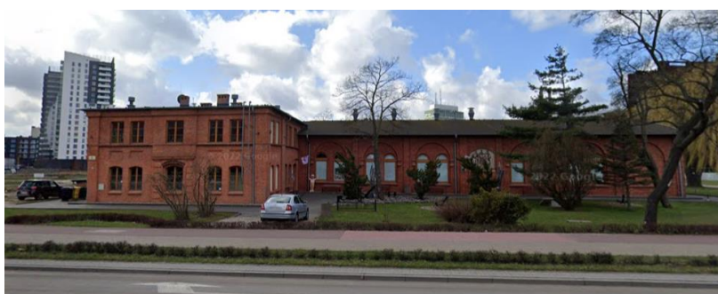
Fig. 4. View of the building from Ks. Jerzy Popiełuszko Street [google.pl/maps, 2024.03.10]
