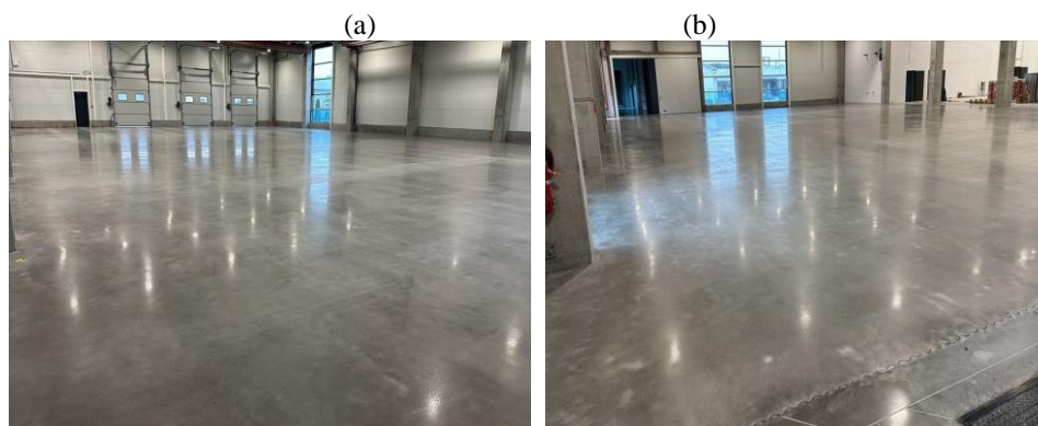
Fig. 13. Concrete industrial floor (Example 3) after regeneration by polishing and impregnation process: a) general view, b) view of pavement treatment in the area of structural expansion joints [38]
