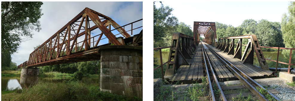
Figure 1. View on railway truss bridge
