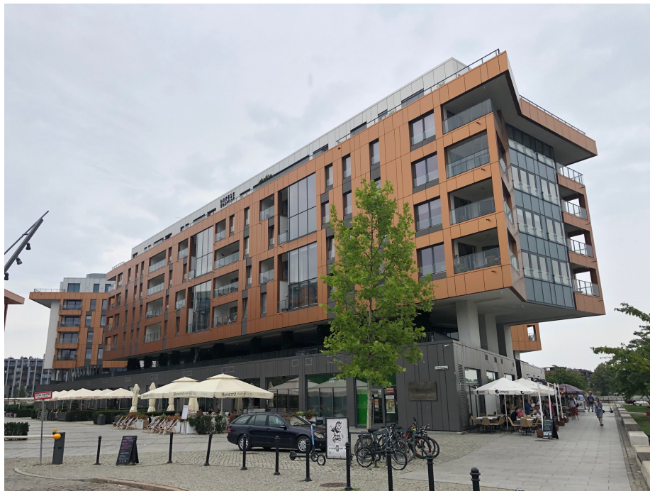
Figure 8.10. Building that the flat is situated in. Source: J. Martyniuk-Pęczek
